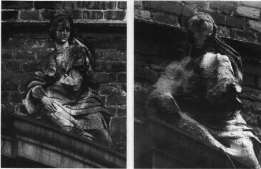
FIGURE 2.6 An example of acid precipitation damage to an outdoor statue. The statue, made of porous sandstone, was created in 1702 as part of the gable of the entrance of the Castle at Hersten, near Rocklinghausen, Germany. The left photo, taken in 1908, shows some stains and the loss of the left hand, but most of the face and right hand were intact after 206 years of exposure. The right photo, taken in 1969, shows the loss of most of the detail of the statue over 61 years [24]. (Reprinted with permission from the Westfälisches Amt für Denkmalpflege.)
